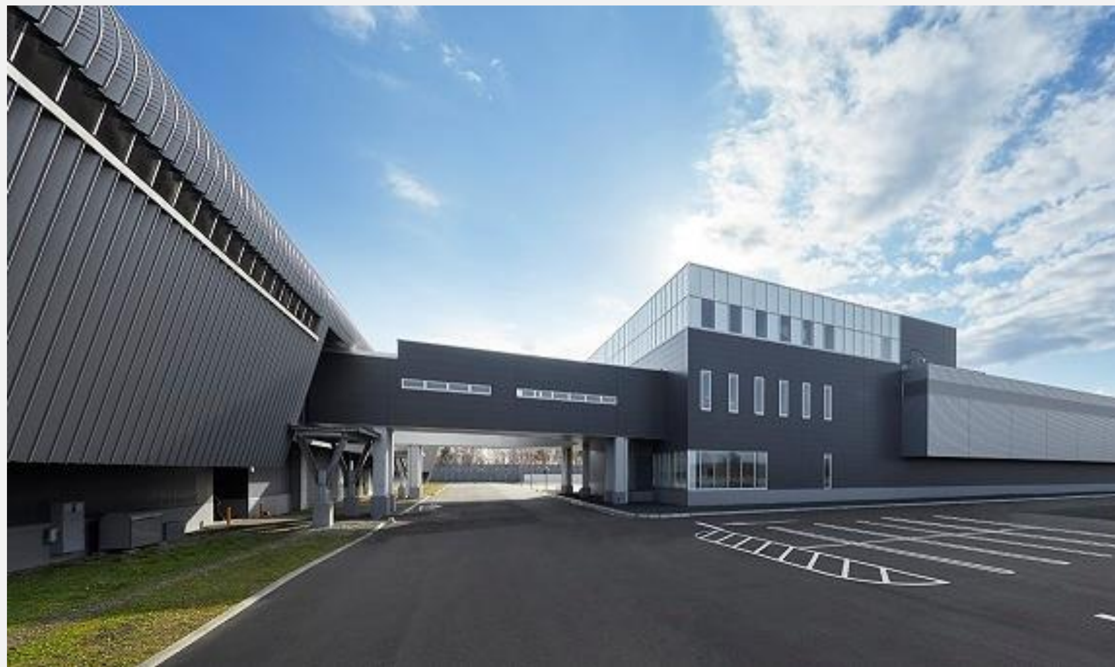
Appearance of Ishikari Dada Center (front: Buildings 3, left: Buildings 1 and 2)
